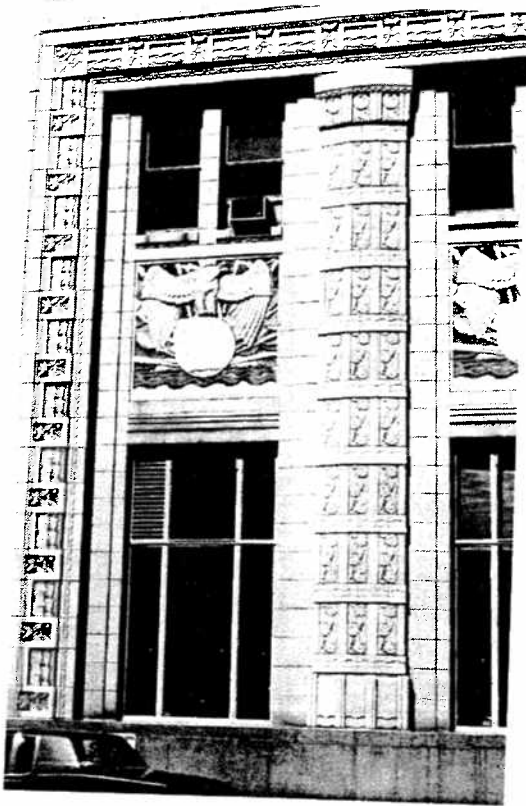
The size of the window openings, as well as their materials and multi-pane arrangements, are integral features of the Laramie State Bank Building. At right, a detail of the entrance-way.
